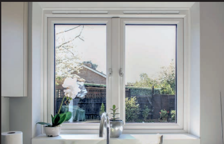
The floating central mullion allows the windows to benefit from the maximum opening without obstruction.
