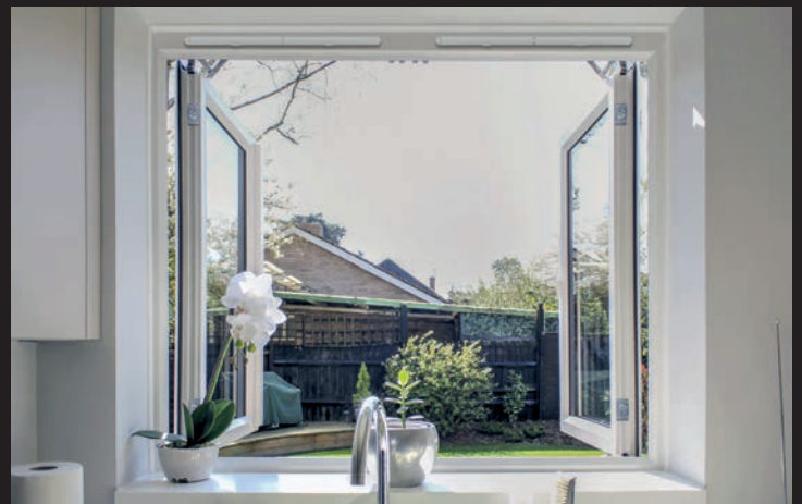
The floating central mullion allows the windows to benefit from the maximum opening without obstruction.
