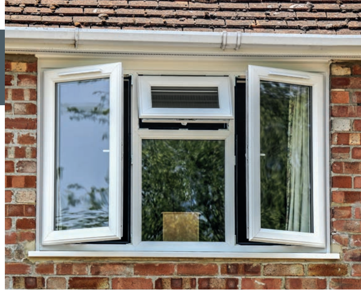
Trickle Vents installed through the window sashes
