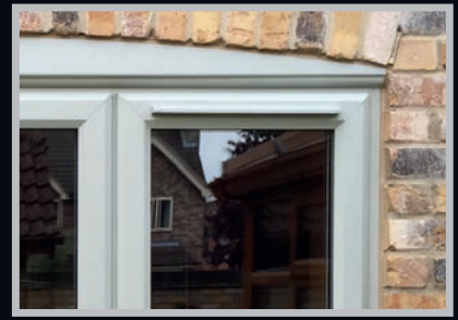
Trickle vent through a Rebated Sash
